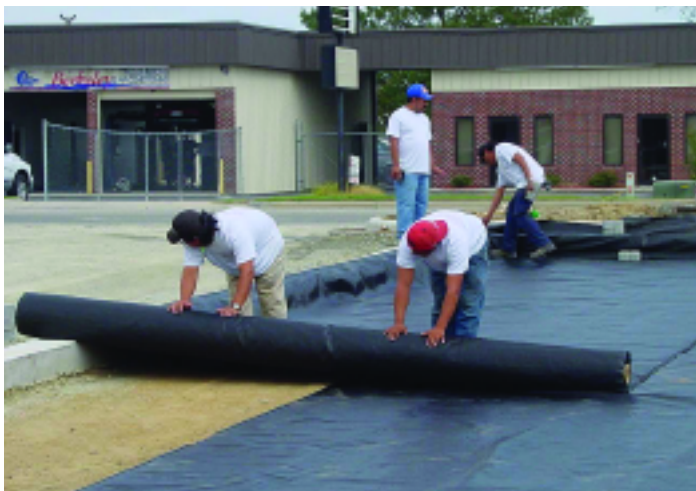
Figure 11. Geotextile is placed over the soil subgrade and lines the bottom and sides of the base.
