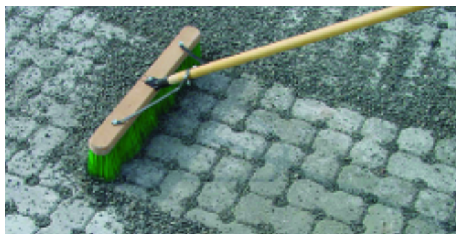
Figure 17. The material used for bedding is also used to fill the openings in the pavers. Powered sweepers are used to distributed stone for large projects. All excess stones are removed from the surface and the pavers are compacted.
