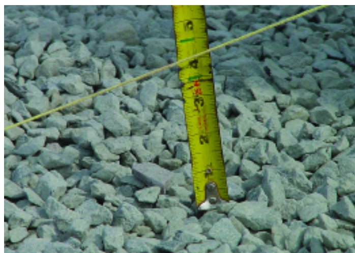
Figure 14. Stone sizes are shown here for a base in a parking lot application in North Carolina. They are compacted and an elevation string line is set for the bedding course and paver installation.
