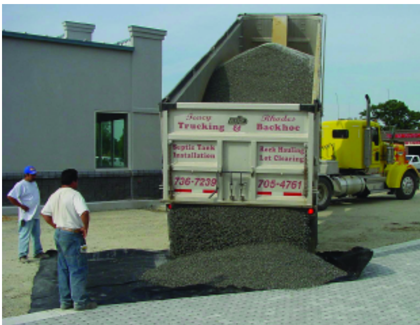
Figure 8. Dumping aggregate on geotextile rather than directly on bare soil helps keep the aggregate from becoming contaminated with sediment.
