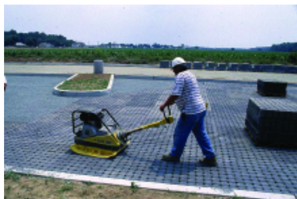
Figure 16. A large plate compactor seats the pavers in the bedding material.
