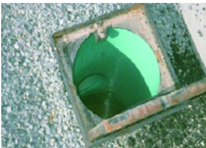
Figure 13. An perforated access pipe at the low side of the pavement allows monitoring of drainage rates.
