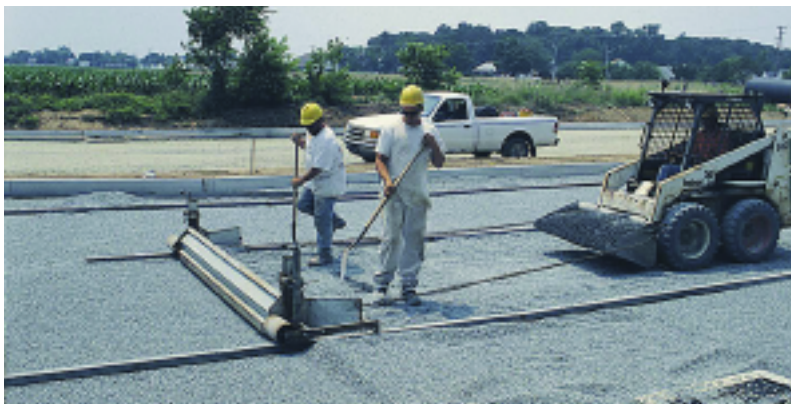
Figure 15. Powered screeding of the bedding layer saves much time compared to hand screeding.
