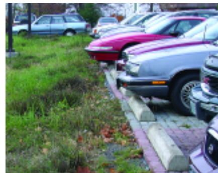
Figure 4. A grass swale receives overflow from this museum parking lot in Portland, Oregon.
