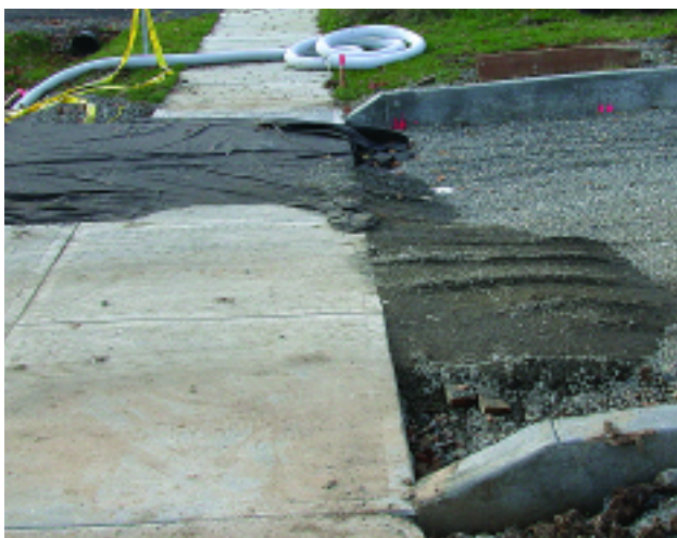
Figure 10. The geotextile on the sidewalk didn't quite make it under the small ramp area made with dense-graded base that rests on installed open-graded base. If it were under the dense-graded material it would help keep some of the fines from contaminating the base. Two or three layers of geotextile would provide a substantial filter of fines.
