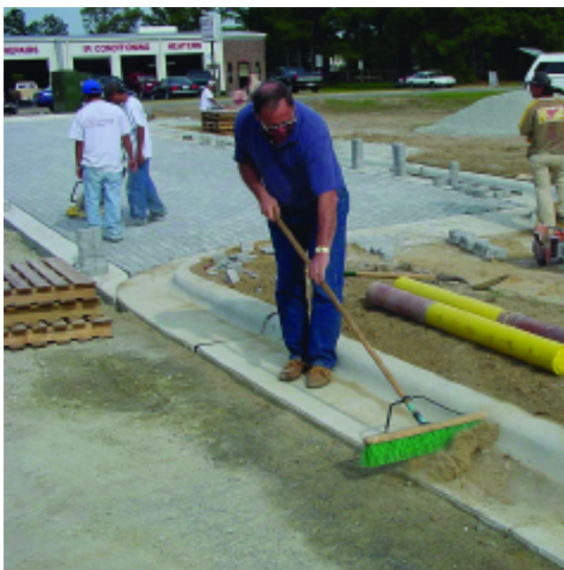
Figure 9. Routine practices such as sweeping away dirt from the pavement while it's under construction will maintain storage capacity in the open-graded aggregate base.
