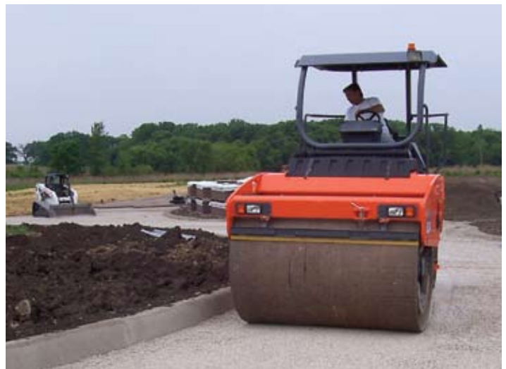
ICPI is evaluating test methods for measuring density and stiffness of PICP open-graded bases using the classic vibratory roller shown here and large plate compactors.
