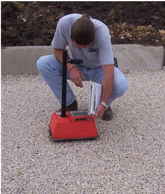
Figure 1. A common site on pavement construction: a technician reads a nuclear density gauge on and PICP project.
