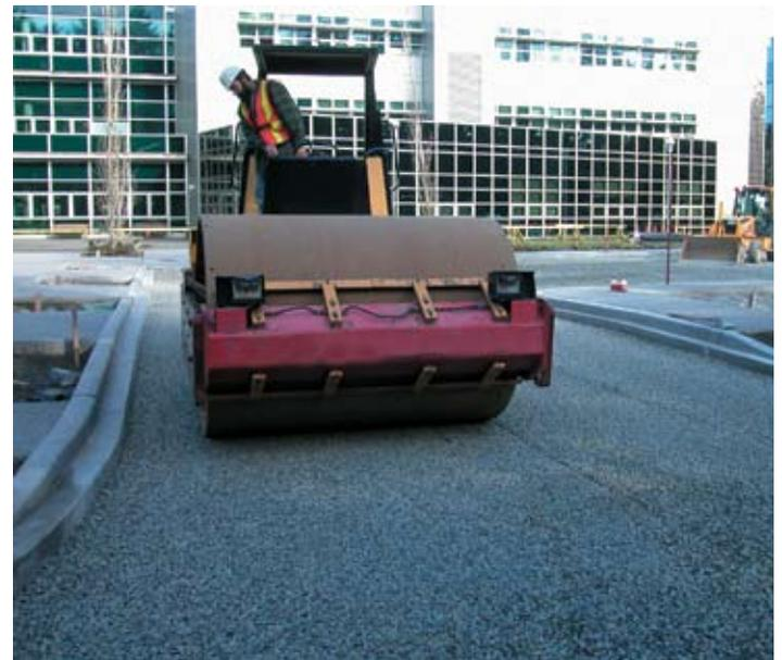
The project specifications called for crushed, open-graded base compaction with initial passes of a roller compactor in vibratory mode, then final passes in static mode.
