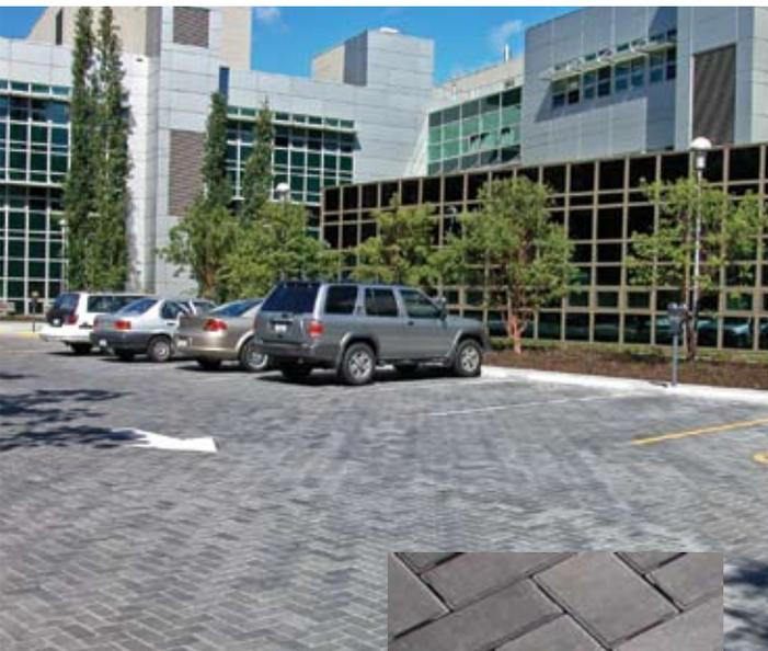
An 8,000 sf (743 m<sup>2</sup>) entrance drop-off and parking lot creates a detention and infiltration for stormwater at the University of Victoria, British Columbia. The fine stone-filled joints infiltrate water from most commonly occurring storms.
