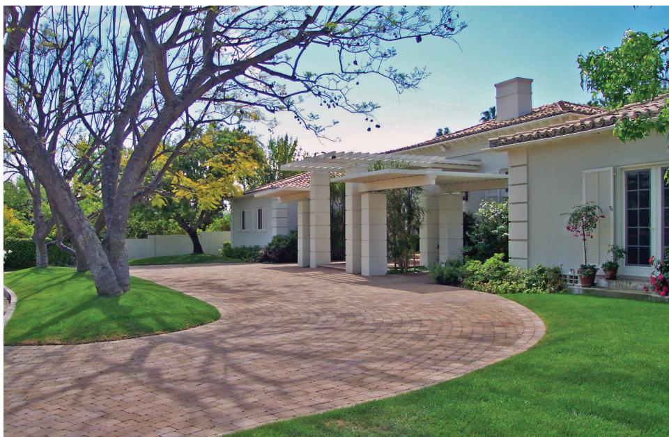
Shown: Quarry Cobble Sand-Stone installed in a running bond pattern.
