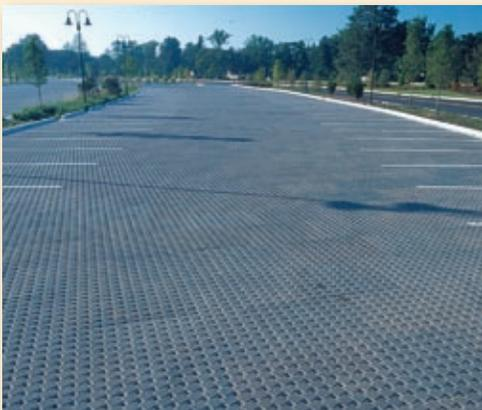
*Morton Arboretum in suburban Chicago expanded its parking facilities with 173,000 sf (16,000 m<sup>2</sup>) of PICPs without building detention ponds. The pavement absorbs rainfall from most rainstorms.*
