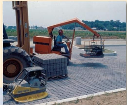
*A clamp on specialized mechanical installation equipment grabs a layer of pavers for placement on the bedding. The pavers are compacted into the bedding layer, the openings and joints filled with the bedding material and compacted again to create interlock among the pavers.*
