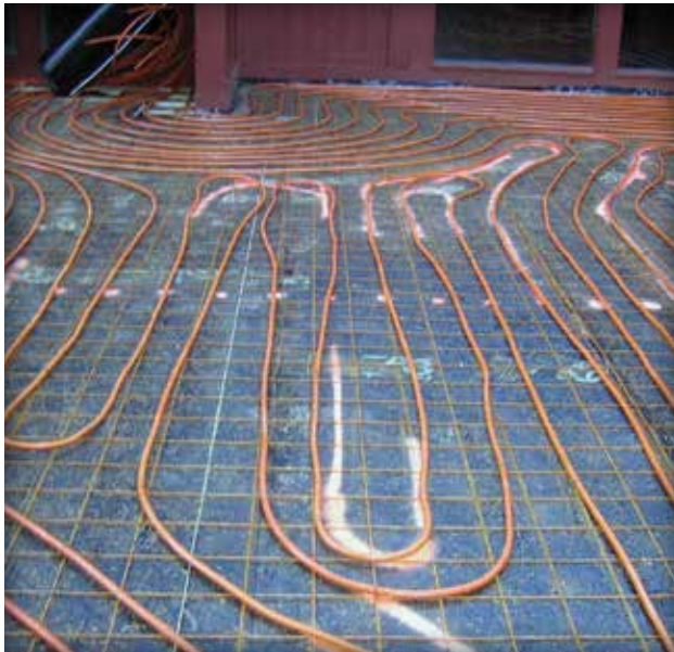
Figure 4. Pipes for a hydronic (liquid) heating system are placed on wire mesh and fastened to it with plastic ties prior to spreading the bedding sand and installing the pavers.
