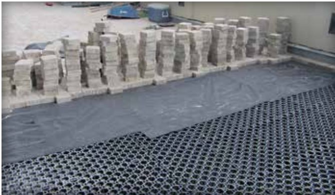
Figure 7. Concrete pavers on geotextile over plastic grids
