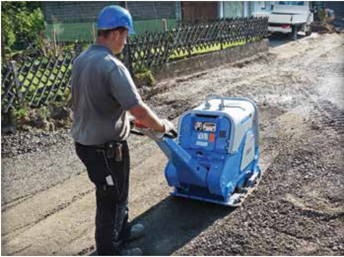
Figure 4. Base compaction with a reversible plate compactor.
