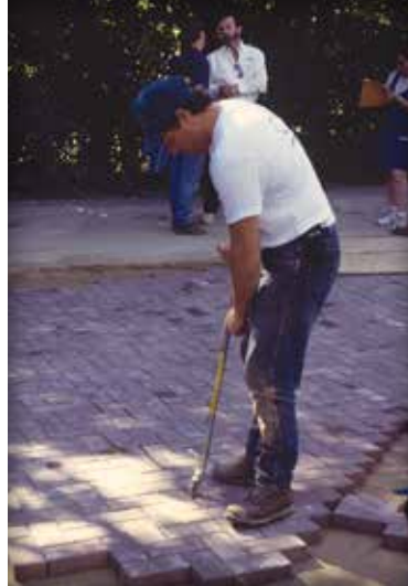
Figure 13. Adjusting joint spacing and alignment.
