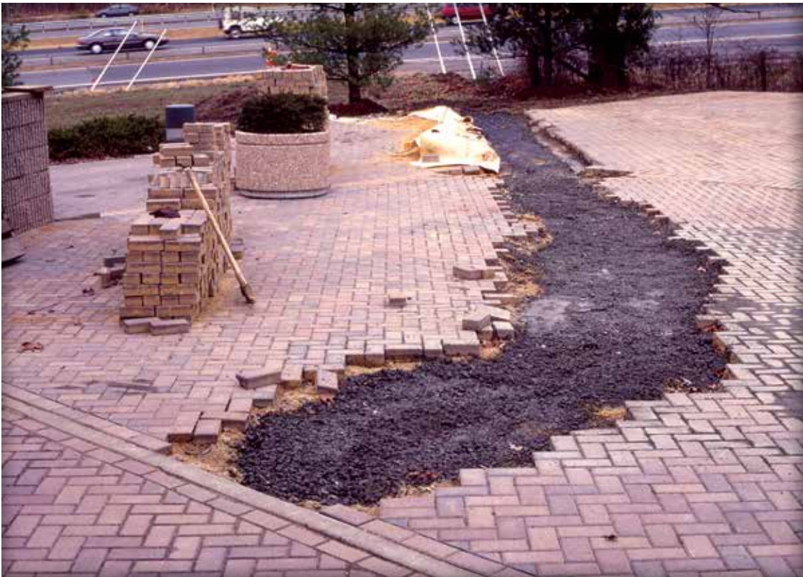
Figure 11. Trench filled with compacted aggregate base. Temporary edge restraints should be used around the opening perimeter.
