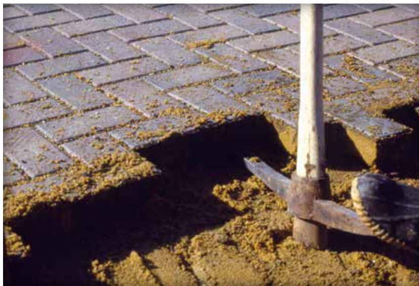
Figure 6. Prying out the remaining pavers
