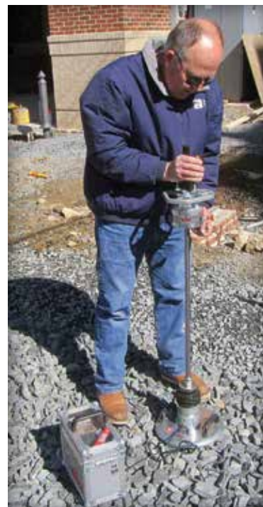
Figure 22. Testing base stiffness using light-weight deflectometer.
