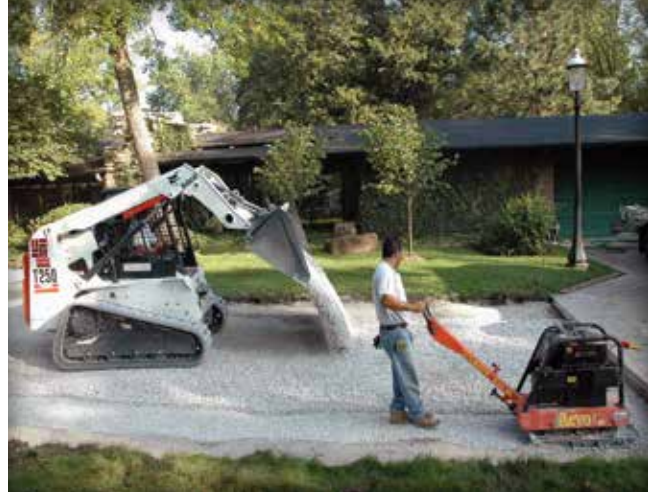
Figure 18. Compacting the berms along the perimeter and the PICP base
