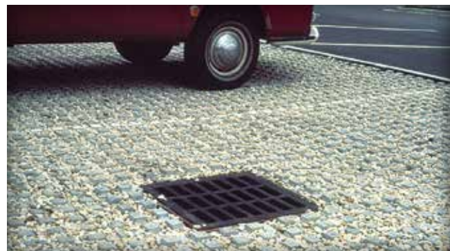
Figure 16. Concrete grids with aggregate in the openings
