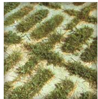
Figure 1. Grids first used in Germany in 1961 for overflow parking were building blocks placed in the ground. They emerged from the need to cool cities and decrease stormwater runoff.
