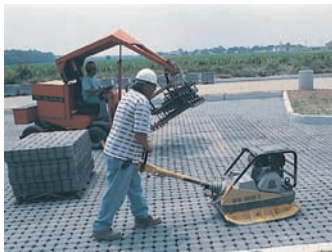
Aggregate base is spread and compacted; pavers are delivered ready to install. After placement of bedding course, joints and/or openings are filled with small aggregate and the pavers are compacted. Joints may be filled mechanically as shown.
