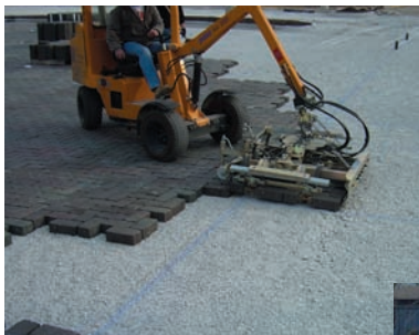
Prepared subgrade for 20,000 sf (2000 m 2 ) Portland, OR street retrofit with PICP
