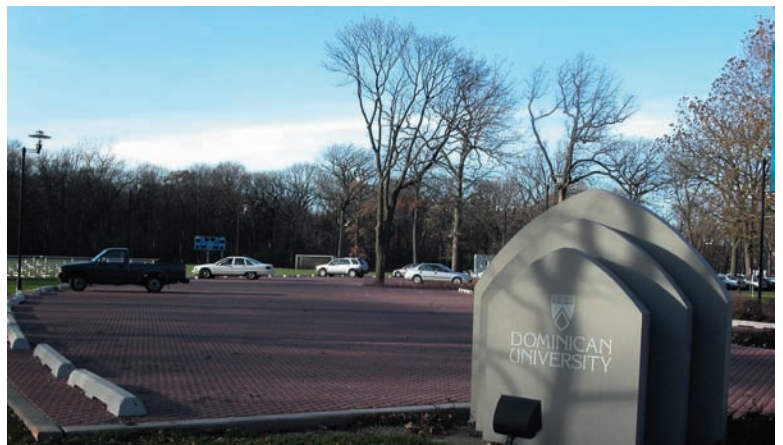
PICP lot eliminates need for detention basin at Dominican University, Chicago.
