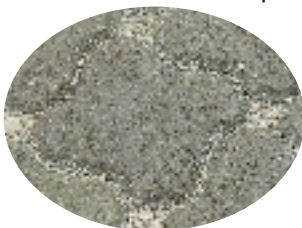
Permeable joint material consisting of small aggregates allows infiltration of stormwater.
