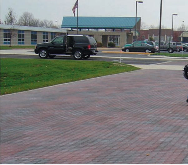
Driveway treats stormwater and reduces runoff at Brentwood School, Plainfield, IN.
