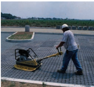
Mechanical installation equipment accelerates construction; typical 5,000 sf (500 m 2 )/ machine/day.
