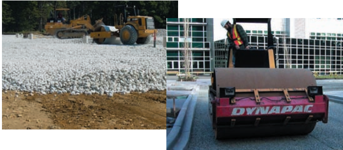
Base construction uses locally available materials.
