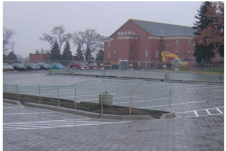
PICP functions as a retention pond and parking lot at the Elmhurst College, LEED® project in Elmhurst, IL, part of an LID sustainable site.
