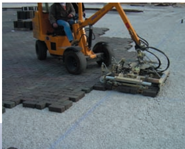
Mechanical installation equipment accelerates construction; typical 5,000 sf (500 m 2 )/ machine/day.
