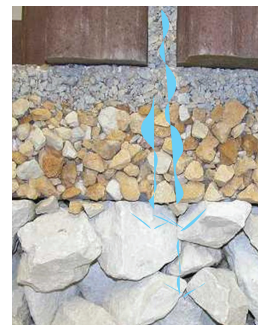
Permeable interlocking concrete pavement (PICP) with open-graded base and subbase for infiltration and storage.
